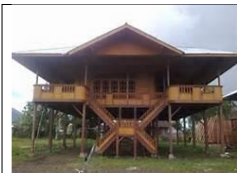
Figure 19. Wooden traditional Minahasa stage house.
